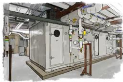
Ordinary Hazard (Group 1) (Mechanical Room)
