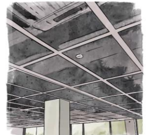
Ceilings (At this stage, finishing pieces for MEP/FP are put in place)
