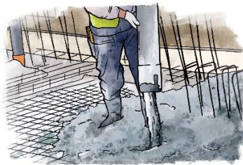
Foundation & Slab Poured (Any floor/slab on grade pouring here)
