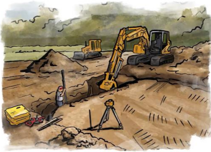
#1 Earthwork (Site Cleared, Graded, Stakes Set)
